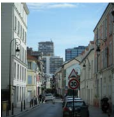
traffic calming measures
